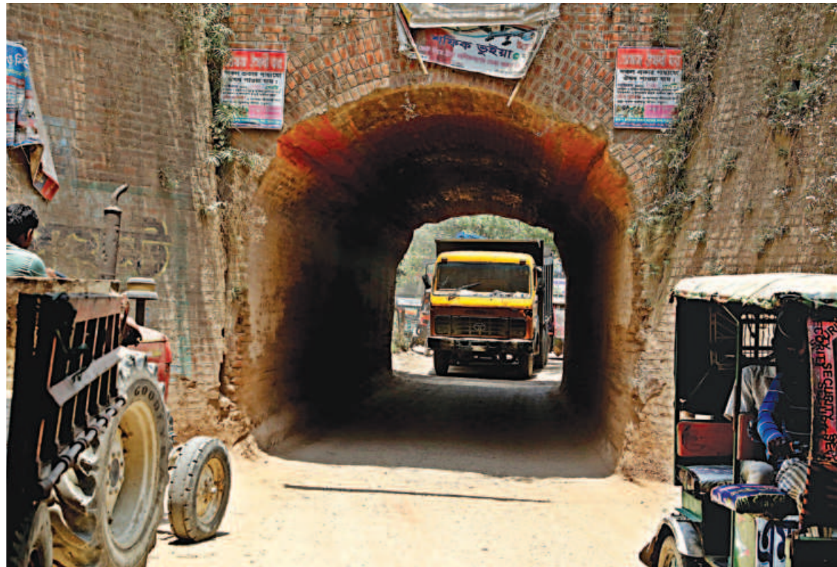
This small tunnel, built in the British era under a rail line, is key for various businesses in Ashuganj of Brahmanbaria to ship in and ship out goods. The old tunnel is getting damaged every day as heavy and tall trucks use the tunnel and scrape its ceiling. The photo was taken recently.
