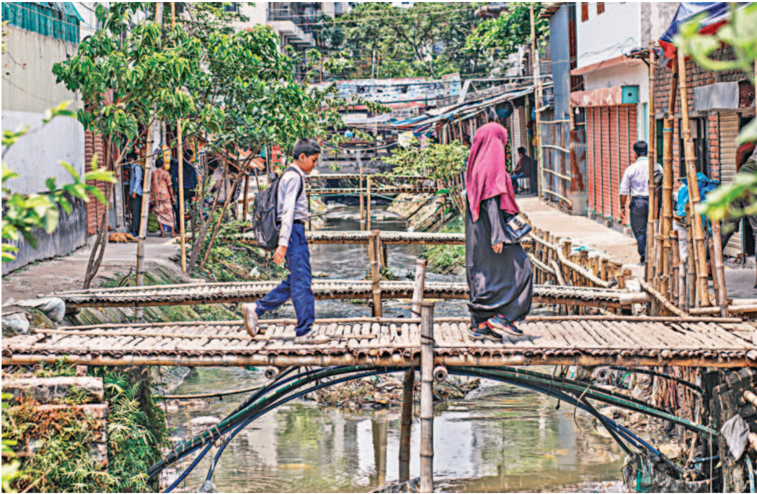
People walk on a makeshift bridge over Kalyanpur canal to go the other side. To save a few minutes, locals have set up multiple such bridges without any safety measures. Meanwhile, the condition of the waterbody continues to deteriorate as garbage dumping and encroachment go on unabated. The photo was taken recently.
