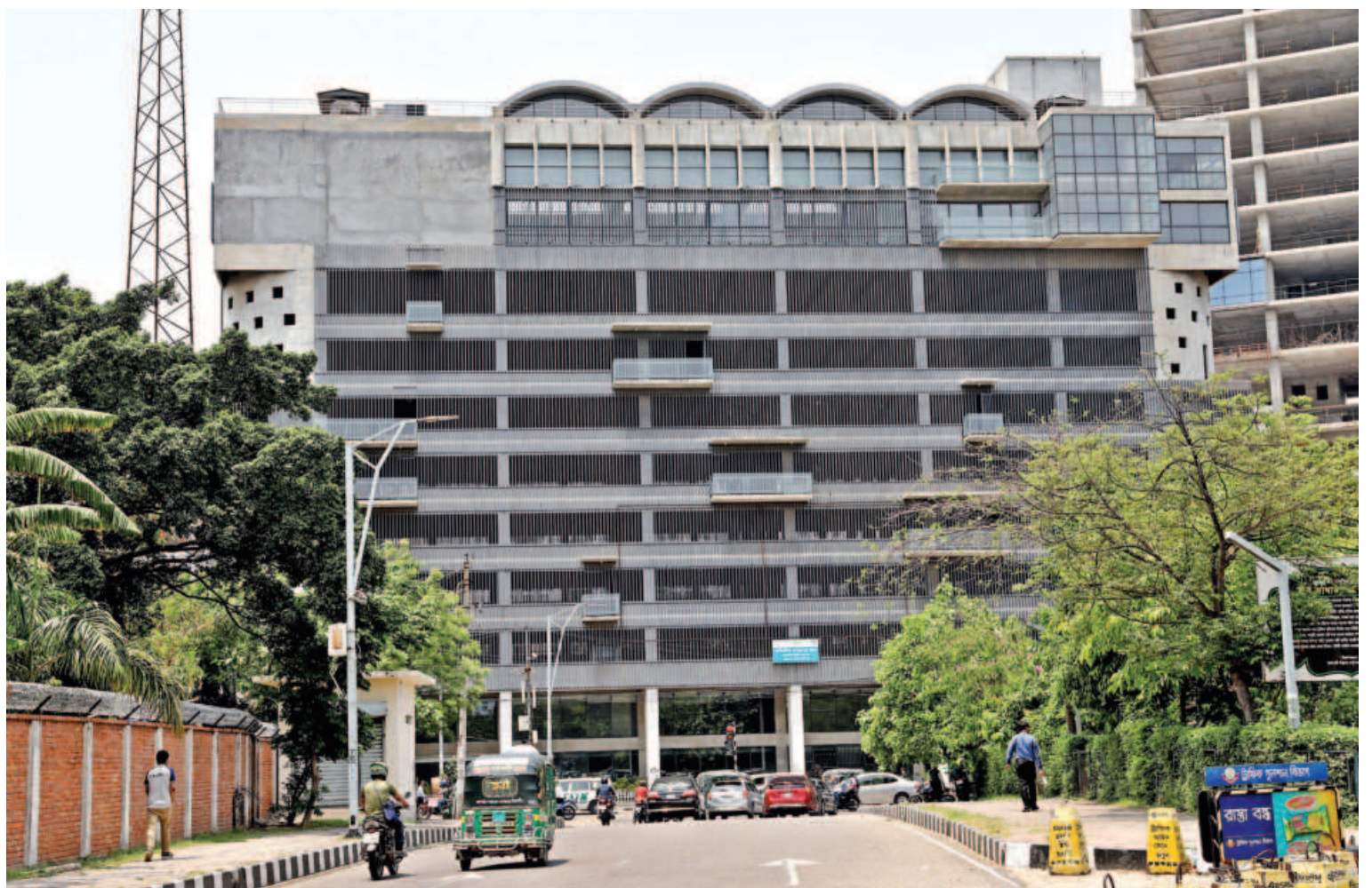
Constructed in 2020, the 10-storey Hatirjheel Car Parking and Management Building of the Rajdhani Unnayan Kartripakkha has been lying vacant for the last three years.
