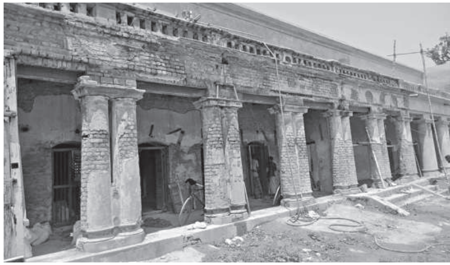
Renovation work for Shilaidah Kachharibari is ongoing.
