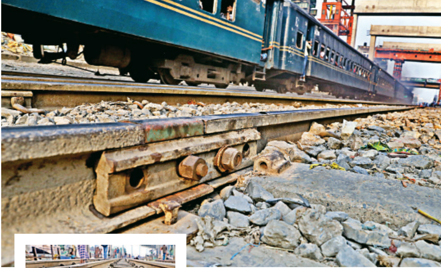
A fishplate, an irreplaceable component in railway tracks, with missing bolts near Malibagh rail crossing yesterday. Meanwhile, multiple clips, another vital part, have been absent from the tracks in Tejgaon railgate area, inset. This photojournalist noticed multiple such bolts and clips missing between the two spots. Such negligence could result in a mishap at any moment.
