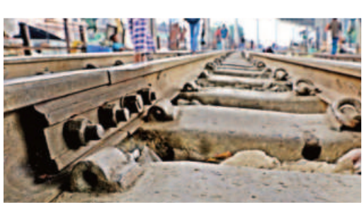
A fishplate, an irreplaceable component in railway tracks, with missing bolts near Malibagh rail crossing yesterday. Meanwhile, multiple clips, another vital part, have been absent from the tracks in Tejgaon railgate area, inset. This photojournalist noticed multiple such bolts and clips missing between the two spots. Such negligence could result in a mishap at any moment.
