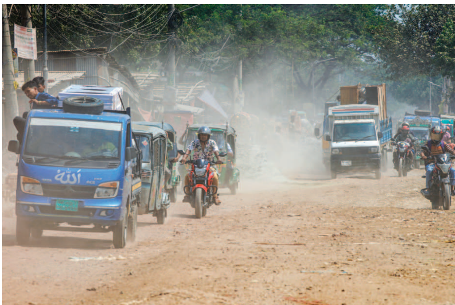
Dust clouds have become regular on the dilapidated Rayerbazar section of the Sadarghat-Gabtolli-Beribadh road, making commute difficult for people in the area. Meanwhile, the road work continues at a snail's pace. The photo was taken yesterday.
