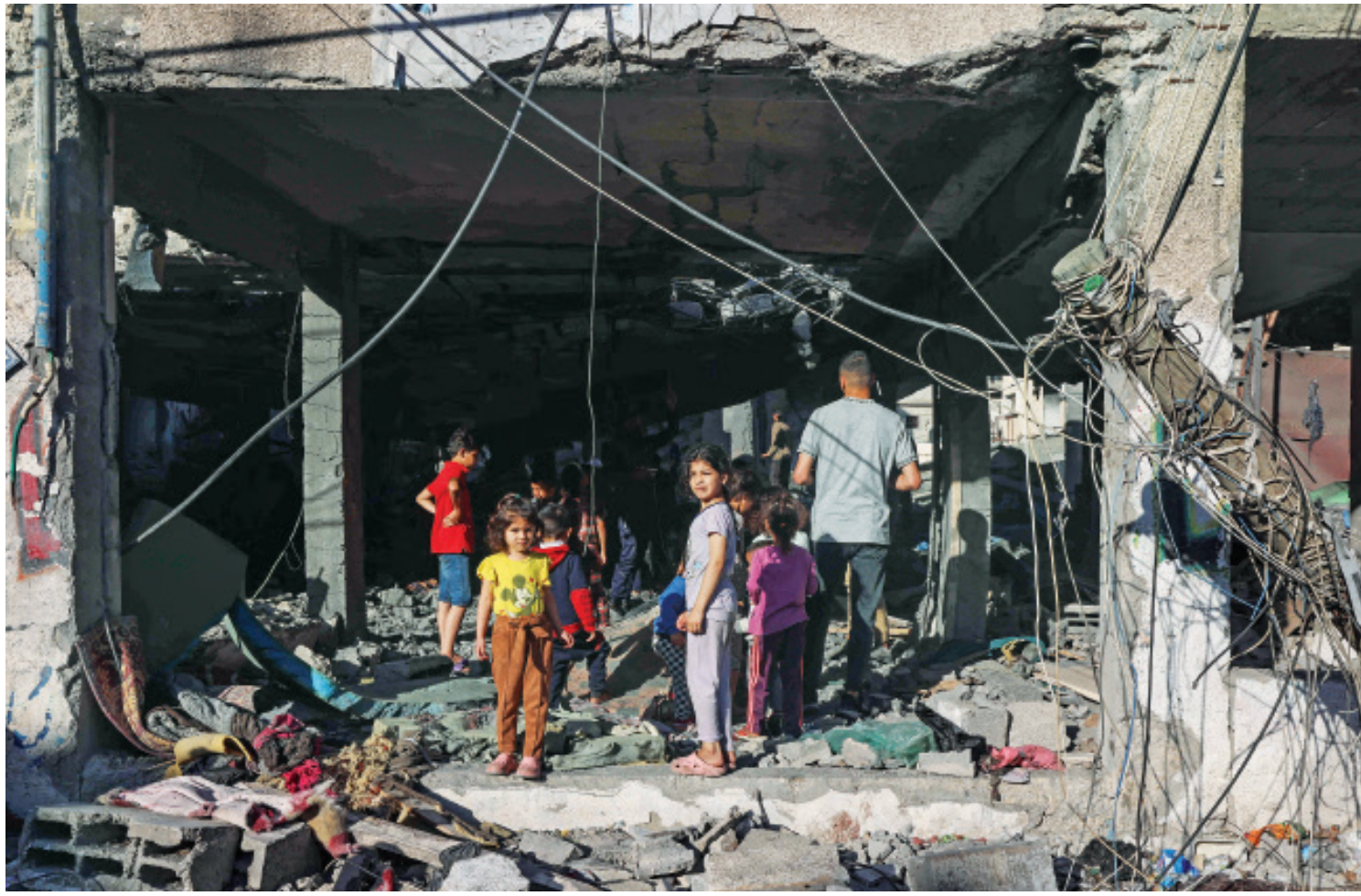
Palestinian children check a building destroyed by Israeli bombardment in Rafah in the southern Gaza Strip yesterday. Israeli media have quoted security sources as saying the long-feared Rafah offensive was due to start this week but the plans have been upended by the Iranian attack.
