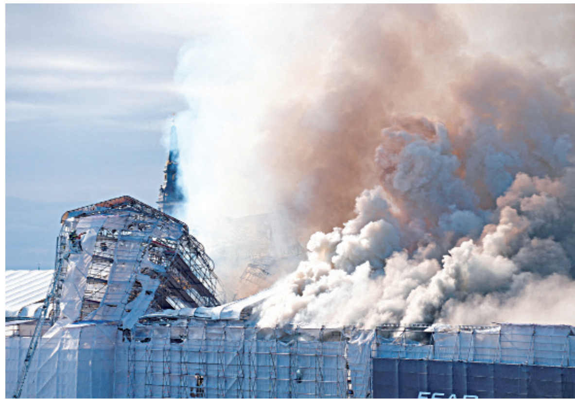
Smoke billows following a fire at the Old Stock Exchange, Boersen, in Copenhagen, Denmark yesterday. There were no reports of injuries, police said, and it was not immediately clear what caused the blaze.
