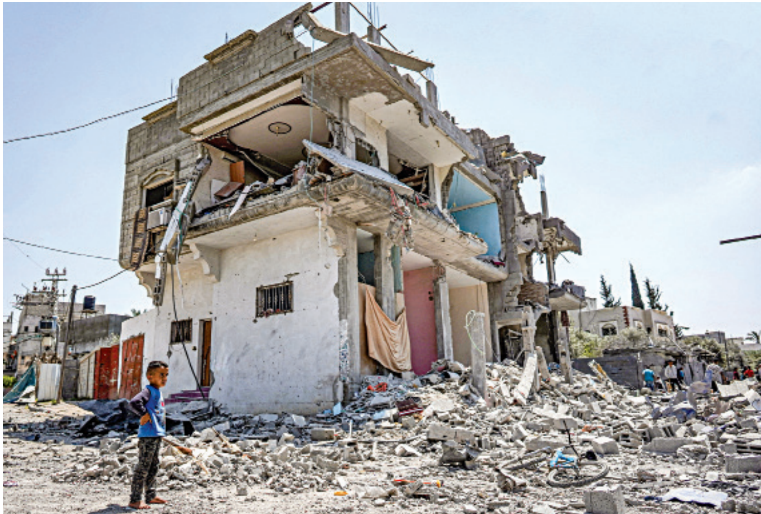
A boy stands by rubble before a heavily damaged building on the eastern side of the Maghazi camp for Palestinian refugees in the central Gaza Strip yesterday amid Israeli offensive in the Palestinian enclave. PHOTO: AFP
