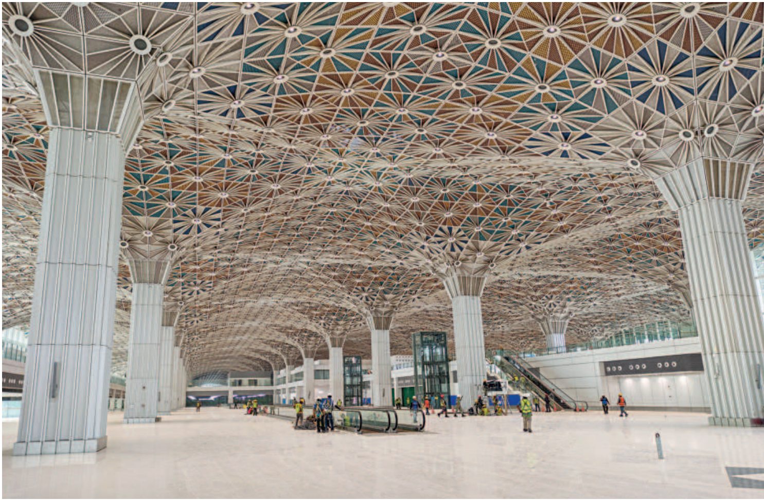
Terminal 3 of Dhaka airport will be handed over to CAAB tomorrow, as it is almost complete. A Japanese company will operate the third terminal, which cost Tk 21,300 crore. The building houses 115 check-in counters, 66 departure immigration desks, 59 arrival immigration and 3 VIP immigration desks. Terminal 3 is expected to be fully ready by October.
