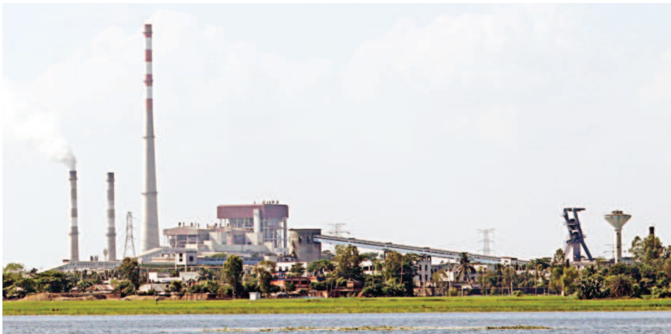
A view of Barapukuria coal-fired power plant in Parbatipur upazila of Dinajpur.
