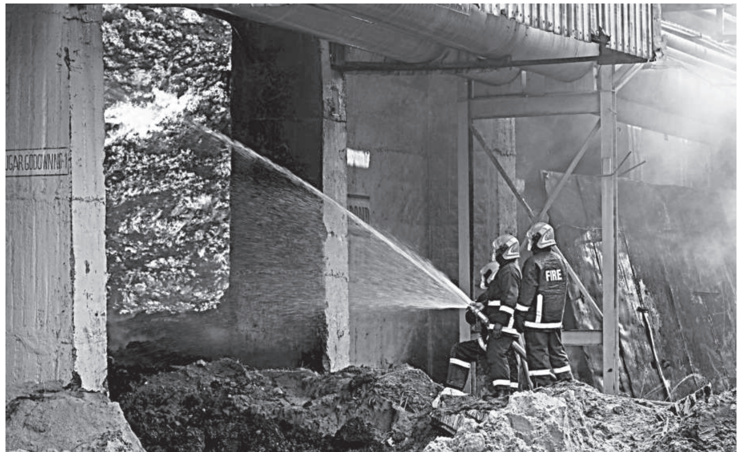
The Bangladesh National Building Code is a crucial document for ensuring fire safety in buildings. However, its implementation remains a significant challenge. PHOTO: RAJIB RAIHAN
