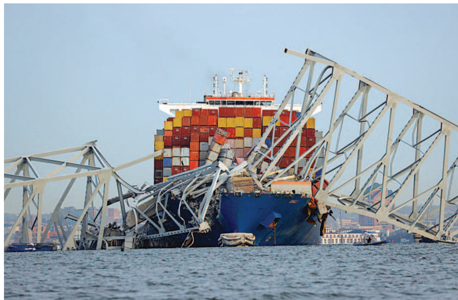
The Dali cargo vessel after it crashed into the Francis Scott Key Bridge causing it to collapse in Baltimore, Maryland yesterday.
