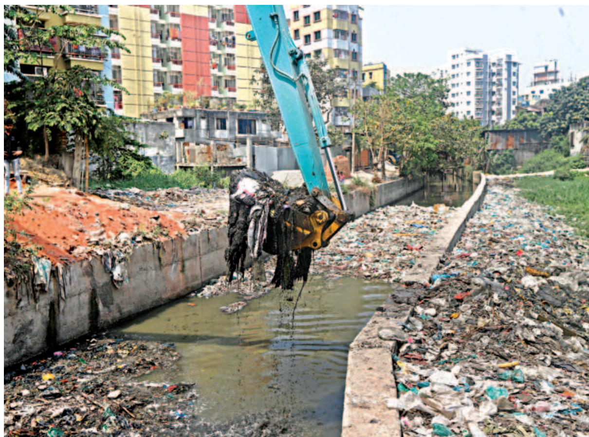
Non-biodegradable wastes being scooped out of the Khilgaon-Basabo canal with a bulldozer in the capital's Madinabagh area yesterday afternoon. The measures were taken to prevent waterlogging in its surrounding areas, ahead of expected rains during summer and monsoon.
