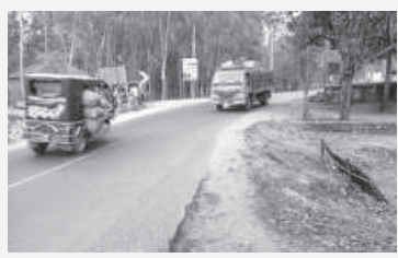
In the last year since March 2023, a total of 43 accidents occurred on the highway, leaving 24 people dead and 48 injured.
