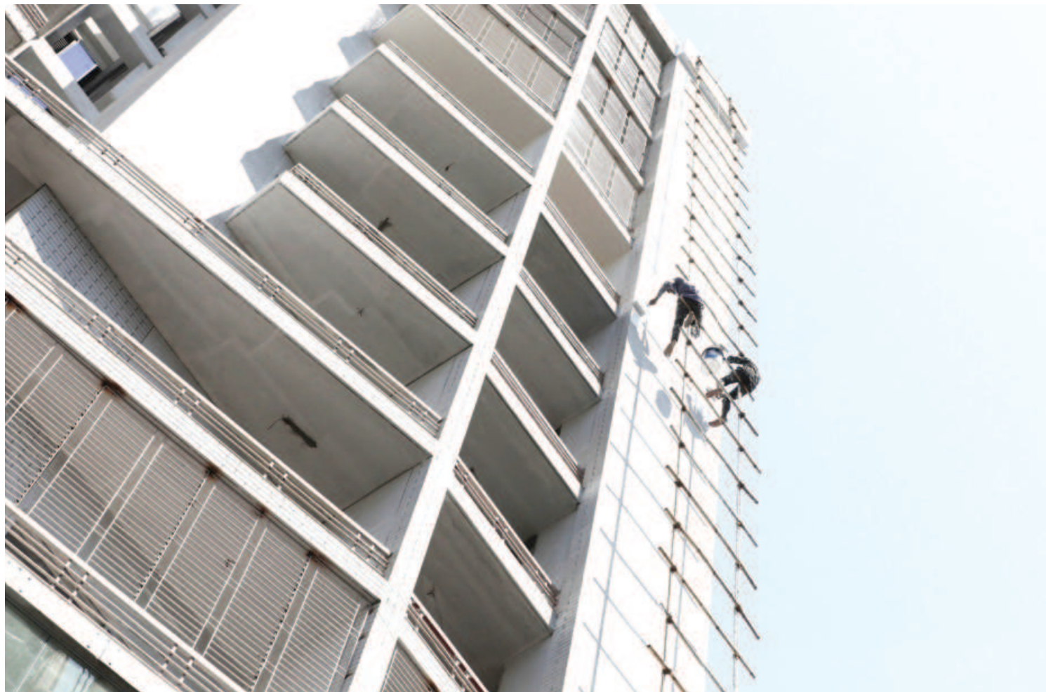
Two men painting a multi-storey building with no safety harness in Notun Bazar area of Mymensingh. According to the Safety and Rights Society, 104 construction workers died at their workplaces in 2022 and falls were the main cause. The photo was taken recently.
