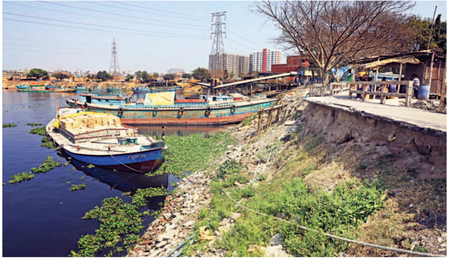
Low water levels in the Turag lay bare the extent of damage done by incoming ships and boats on the embankment in the capital's Gabtoli. In the absence of barriers, vessels often crash against the banks when the river is full, causing erosion and raising the possibility of the adjacent walkway to cave in. The photo was taken yesterday.
