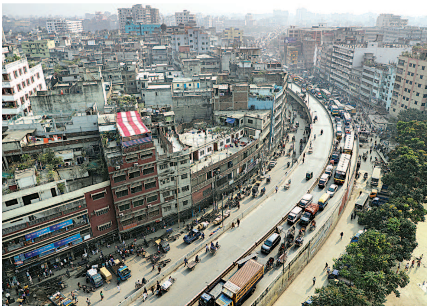
The Buriganga-2 bridge, otherwise known as Babu Bazar bridge, saw long tailbacks throughout yesterday as the Buriganga-1 bridge, or the Postogola bridge, has been shut down for repair work. The work, which started on February 22, will continue till March 8 and the bridge, which connects Dhaka to 21 districts, will be closed for days in different phases.
