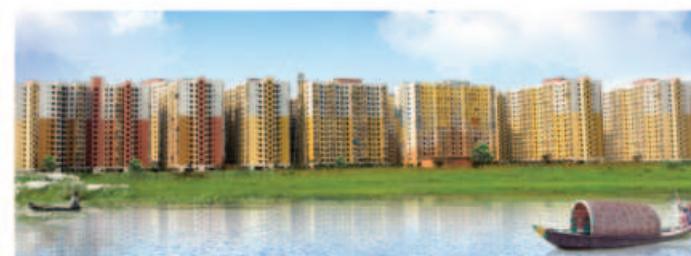
2000 First satellite township of Bangladesh, Lake City Concord was built at Khilkhet with over 4000 apartments, shopping & commercial blocks, school, mosques, landscaped gardens and all other lifestyle facilities
