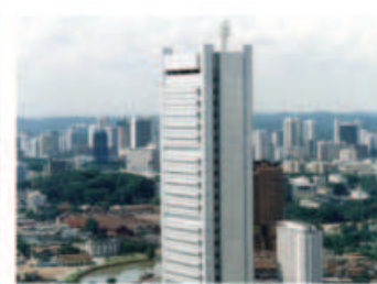
1984 Constructed Telecom Building in Singapore
