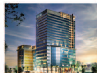
2006 Introduced Top Down Construction Method in Bangladesh through construction of WTC in Chattogram
