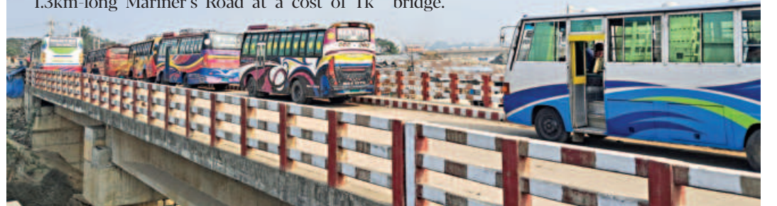
Due to a lack of approach roads, the two-lane bridge over Rajakhali canal in port city's Kotwali area is now being used for parking buses.
