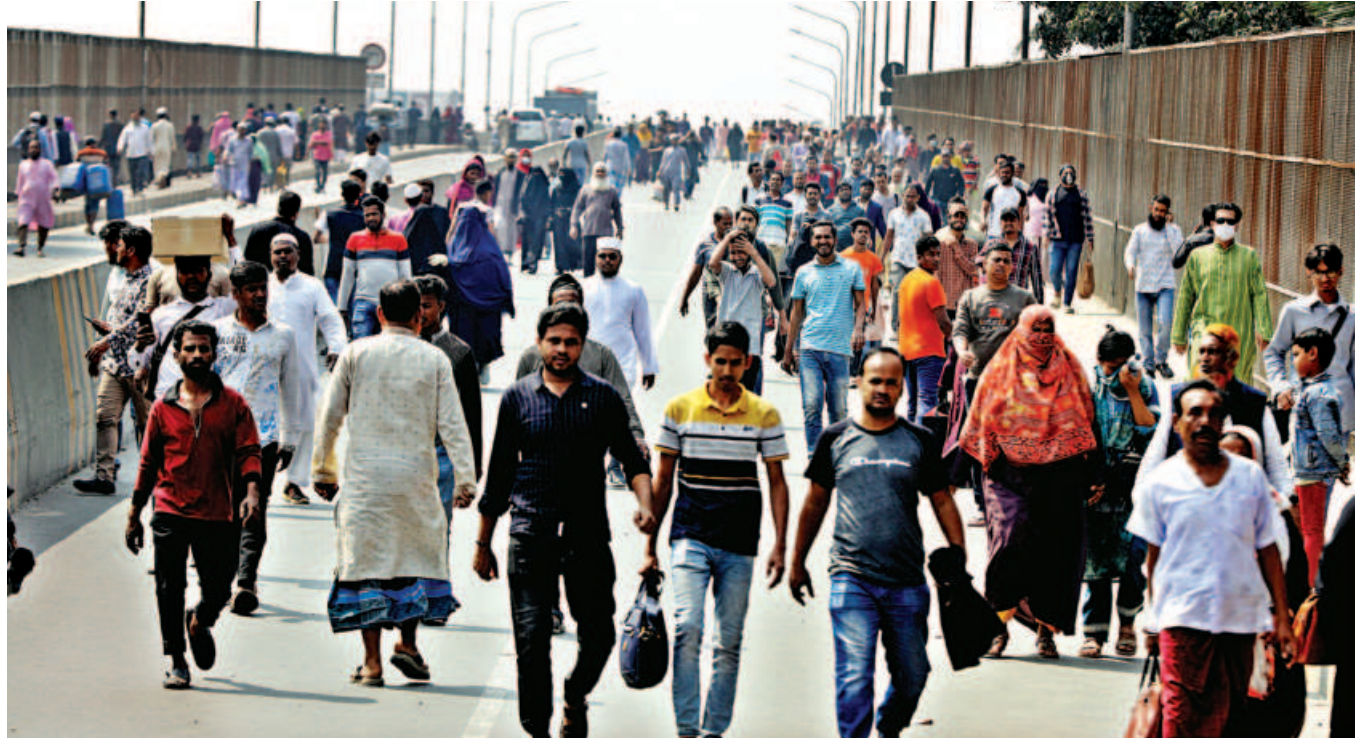
People walk across the First Buriganga Bridge in Postagola yesterday as the bridge has been closed to traffic since midnight Friday. The Road Transport and Highways Division announced that the bridge would be closed in phases until March 8 for restoration work.
