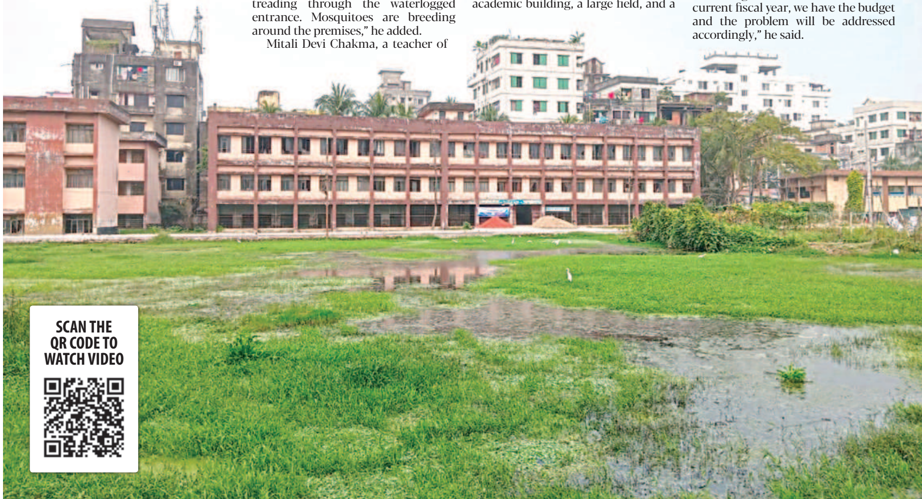
The Government Teachers' Training College at Chawk Bazar remains waterlogged throughout the year. According to students, this problem has been persisting for over five years now. PHOTO: STAR
