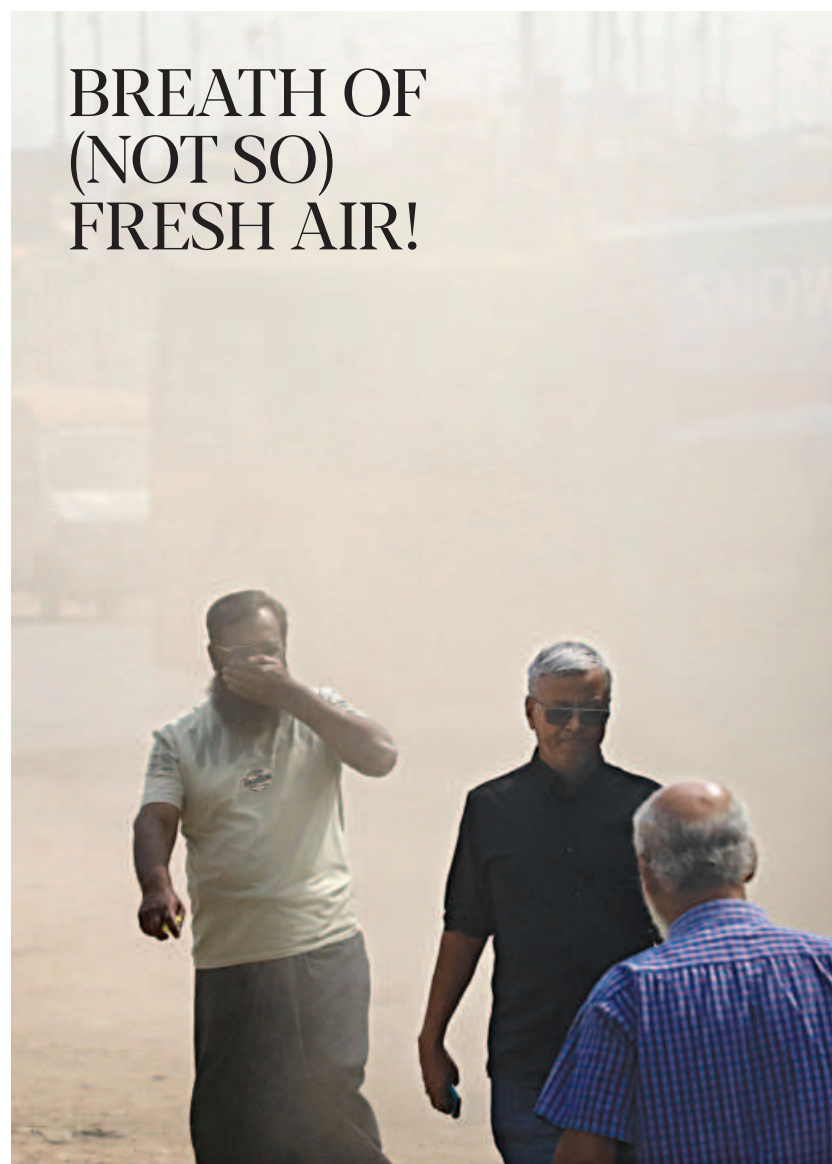
PHOTO: PALASH KHAN Covering his nose, a man hurries away from a gust of dust on the Dhaka-Aricha Highway in Savar's Amin Bazar area yesterday. Dust from road-digging as well as unplanned and uncoordinated construction works continue to plague this stretch of the road, posing health risk to commuters.
