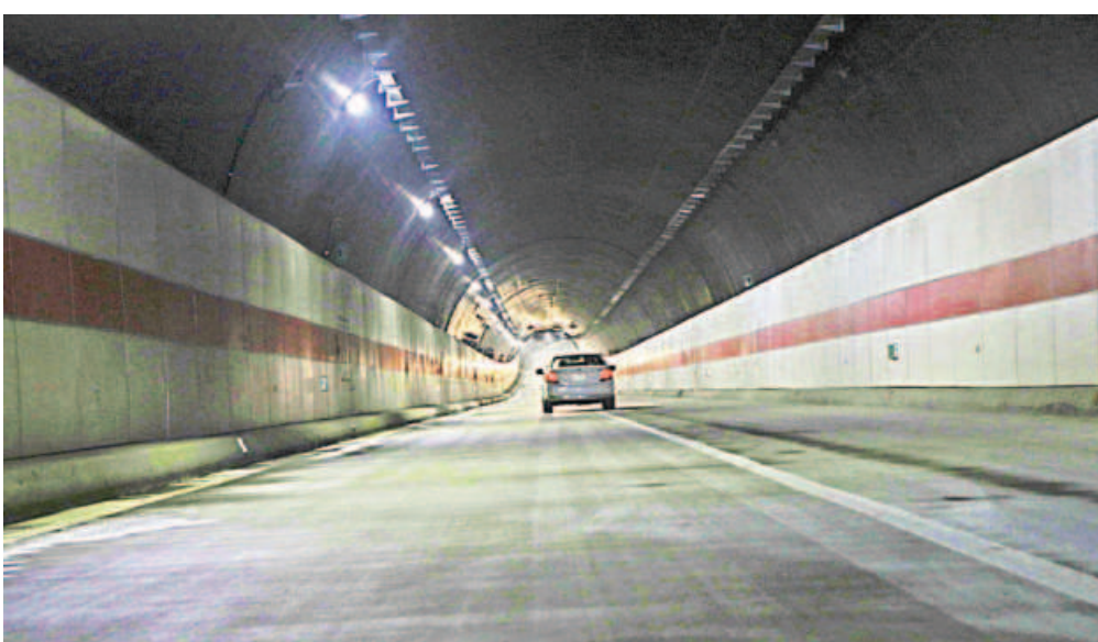
An inside view of the Bangabandhu Sheikh Mujibur Rahman Tunnel under the Karnaphuli river in Chattogram.
