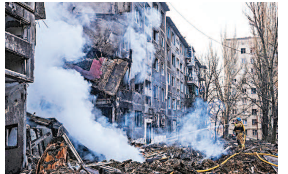
A firefighter works at the site of a residential building destroyed in a Russian missile attack, in Selydove, Donetsk region, Ukraine yesterday. PHOTO: REUTERS
