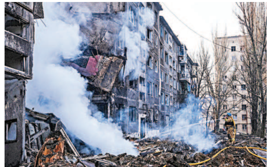
A firefighter works at the site of a residential building destroyed in a Russian missile attack, in Selydove, Donetsk region, Ukraine yesterday. PHOTO: REUTERS
