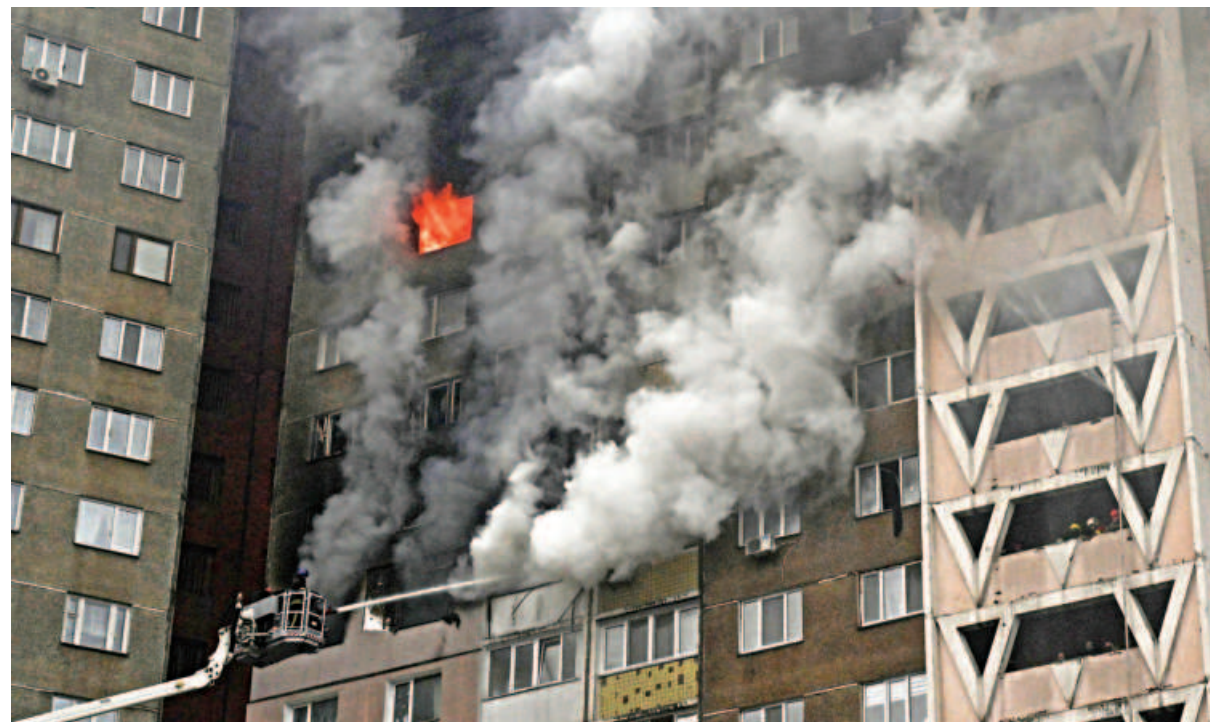
Firefighters work at a site of a building damaged during a Russian missile strike, amid Russia's attack on Ukraine, in Kyiv yesterday. Russia unleashed missile and drone strikes on Kyiv and other Ukrainian cities during morning's rush hour, killing five people, wounding more than 30. PHOTO: REUTERS
