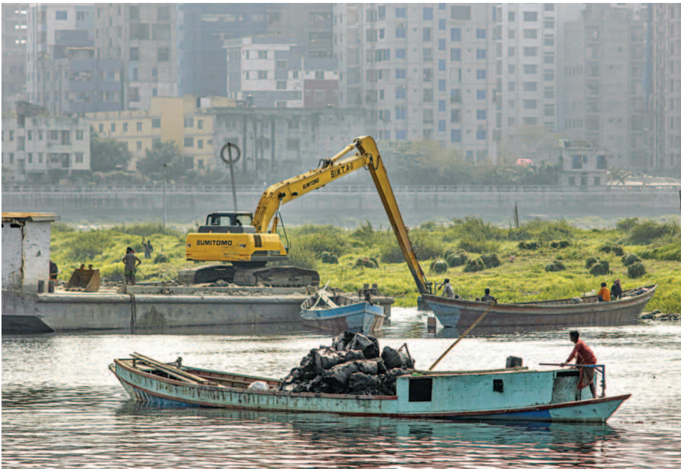
A BITWA excavator extracting mud from the riverbed of the Turag near Dhaka's Gabtoli to improve navigability and widen the channel. Cargo vessels carry the mud to different areas to fill up low-lying land. The photo was taken on Saturday.
