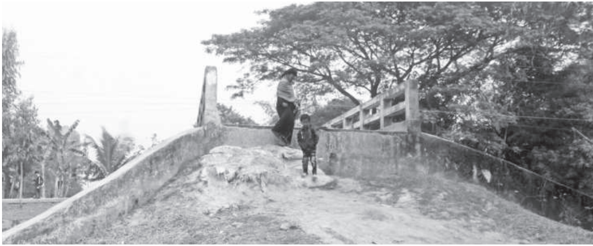
For over eight years, residents of Kadamtara at Habiganj's Bhagulipara continue to suffer as an eight-metre-long bridge over the Dhulia canal remains inaccessible due to the absence of approach roads. PHOTO: STAR
