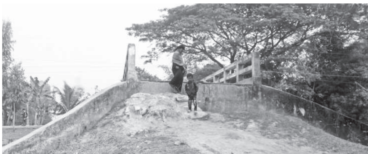
For over eight years, residents of Kadamtara at Habiganj's Bhagulipara continue to suffer as an eight-metre-long bridge over the Dhulia canal remains inaccessible due to the absence of approach roads. PHOTO: STAR
