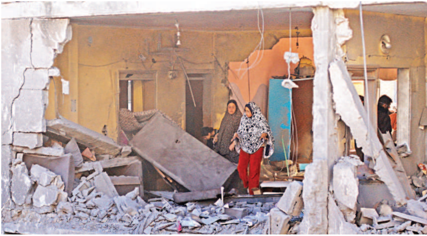
Palestinians inspect the site of an Israeli strike on a residential building in Rafah in the southern Gaza Strip yesterday. PHOTO: REUTERS
