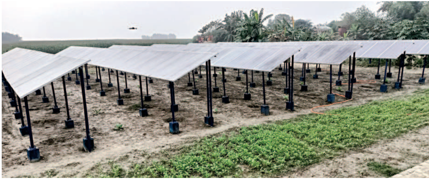
An array of 192 solar panels that generate about 57.6 kilowatts of electricity each day have been installed at a remote char called Ghughumari in Ulipur upazila of Kurigram. Established under an initiative of Standard Chartered Bangladesh and Friendship, the "Solar Village" is bringing power to about 150 homes in the area.
