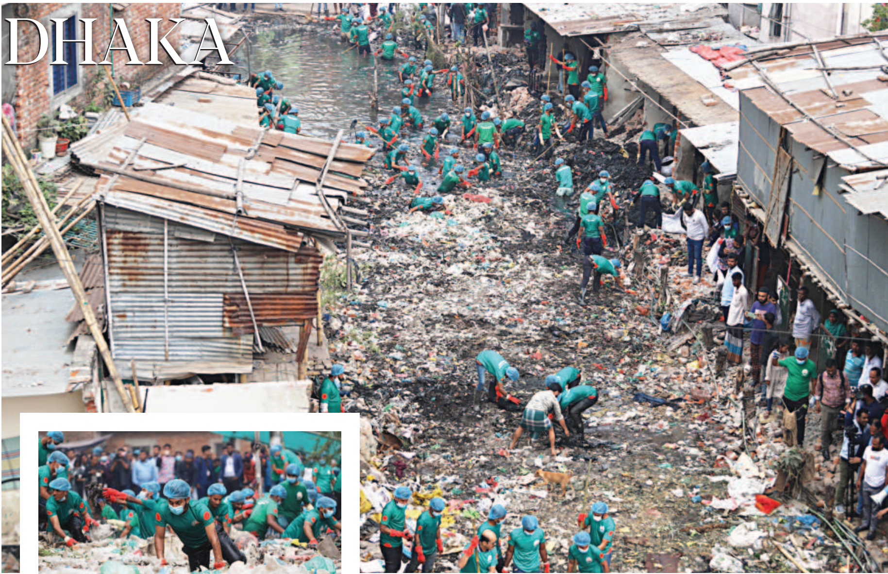
Around 1,200 volunteers of BD Clean along with DNCC began cleaning Mirpur's Paris Canal yesterday. The initiative hopes to restore this canal to its former glory, removing all illegal structures and wastes that have left the waterbody on the brink of death.
