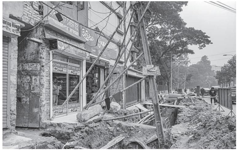
An electric pole tilts towards a shop as workers dig up a significant portion of the Mansur Ali Sarani in the capital's Moghbazar for drainage works. Though supported by bamboo canes, the pole remains in a precarious position and may fall any minute, damaging the shop entirely. Besides, pedestrians are also forced to walk on the street, risking lives, as the work goes on at a snail's pace. The photo was taken recently.
