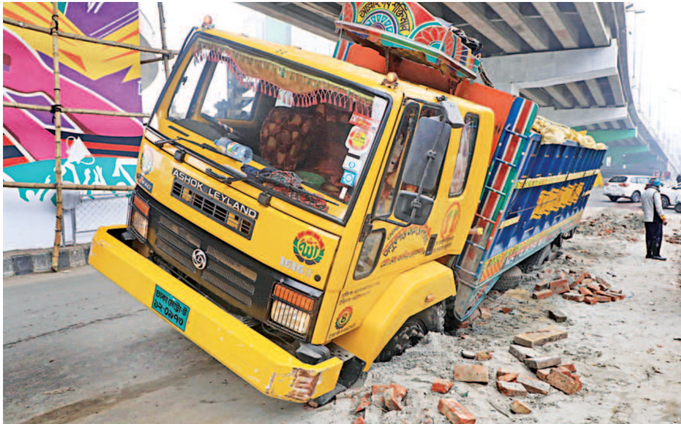
A lorry stuck near the FDC intersection in the capital around 8:30am yesterday. Lanes of the street had not been paved after the asphalt was ripped up for the installation of underground cables.
