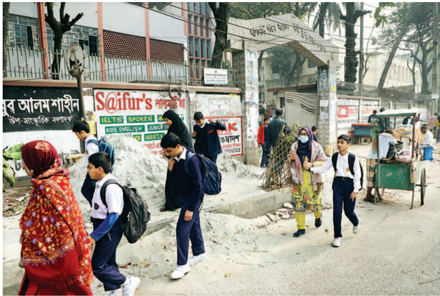
Schoolchildren and pedestrians are forced to walk on the street near the gate of Dhanmondi Government Boys' High School in Dhaka as people tasked with repairing the pavement have left a pile of sand there. The photo was taken yesterday.
