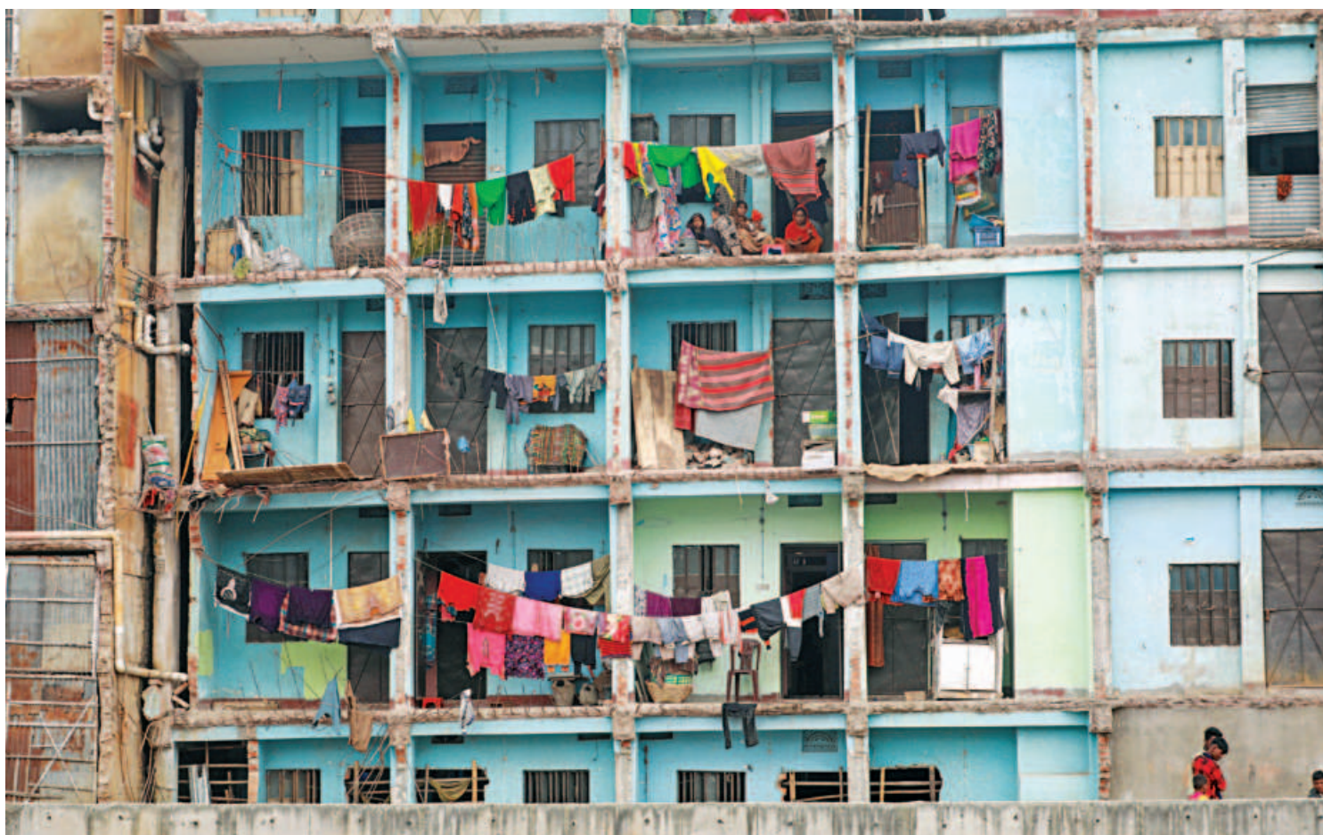
Many families, even with small children, living precariously in a half-demolished building in Chattogram city's Tulatali area. As it was constructed illegally on the banks of a canal, the encroaching portion was demolished during a drive around nine months ago. However, the remainder of the building was not repaired, posing risks to all those living in it. The photo was taken yesterday.
