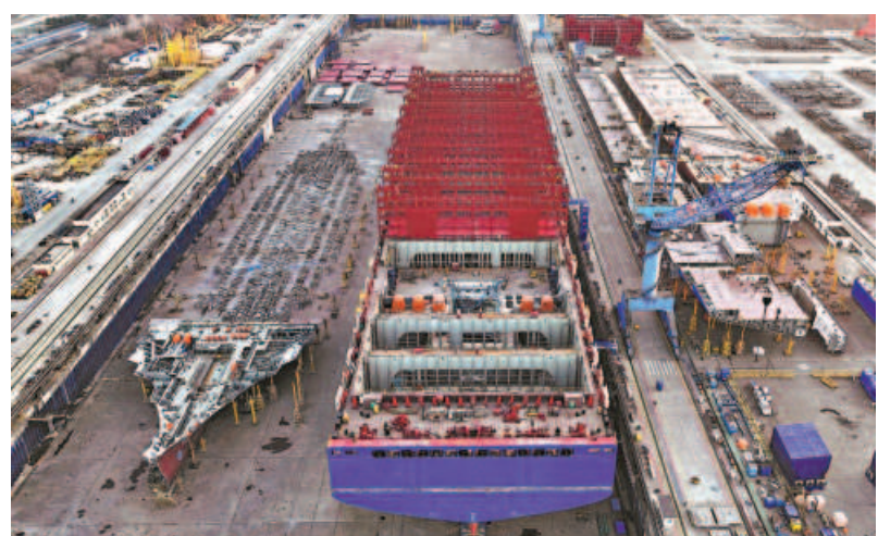
A vessel is under construction at a shipyard in Yangzhou, Jiangsu province, in China.
