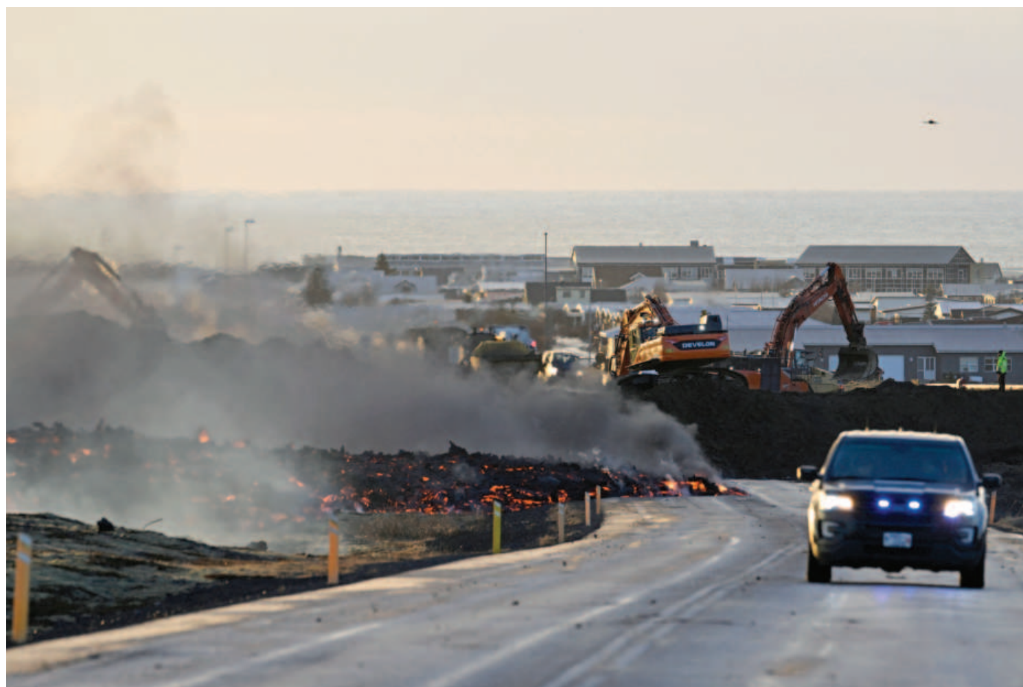
Emergency personnel use diggers to fill in the last hole in a protective wall trying to prevent flowing lava to reach the centre of the southwestern Icelandic town of Grindavik after a volcanic eruption yesterday.
