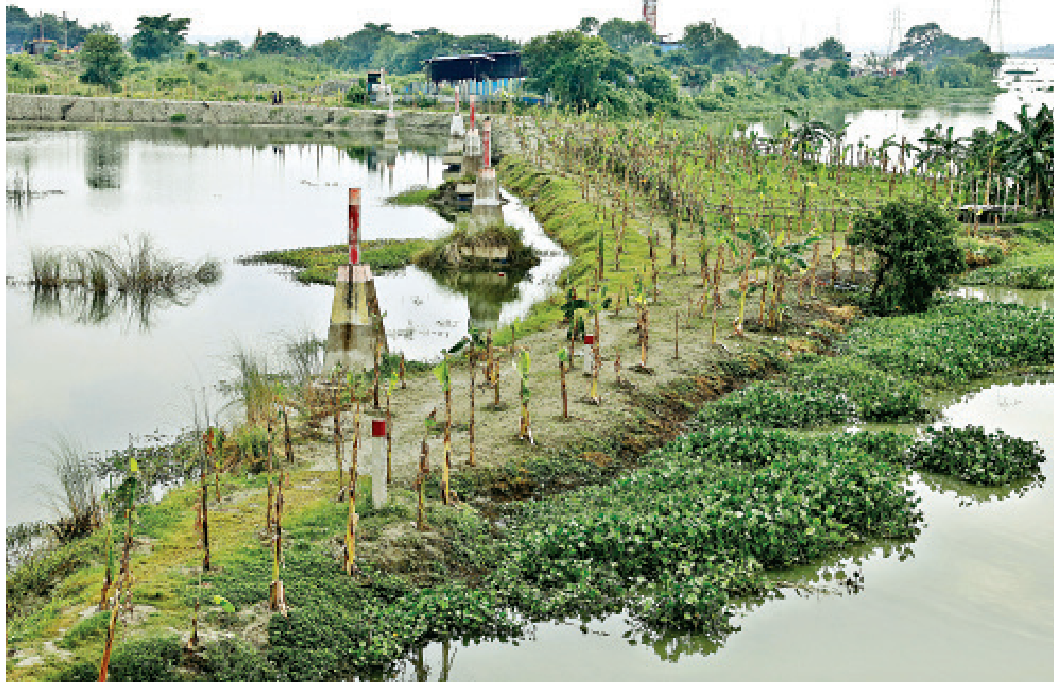
Ignoring the demarcation pillars set up by the BIWTA, encroachers have illegally filled up a portion of the Turag, near the Birulia-Ashulia highway on the outskirts of the capital, and made their own garden there. The photo was taken from the Birulia bridge recently.
