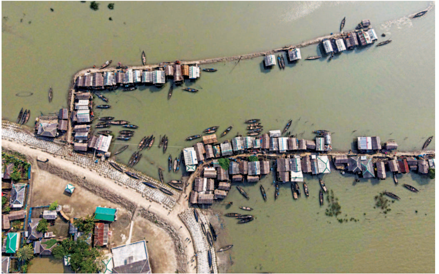
THE HANGING VILLAGE ... After losing everything to river erosion, the locals of Kalabagi in Sutarkhali union of Khulna's Dakop upazila -- a village bordering the Sundarbans -- have had to build makeshift bamboo homes over the river Shibsra. This cluster of dwellings is now known as "Jhulantapara" (the hanging village). Living precariously, people there are also deprived of safe food and water, along with hygienic toilets or medical facilities. PHOTO: HABIBUR RAHMAN
