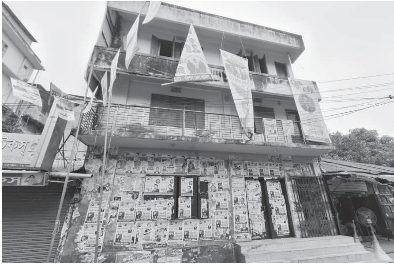
A deserted BNP central office on Barishal city's Nagar Road.
