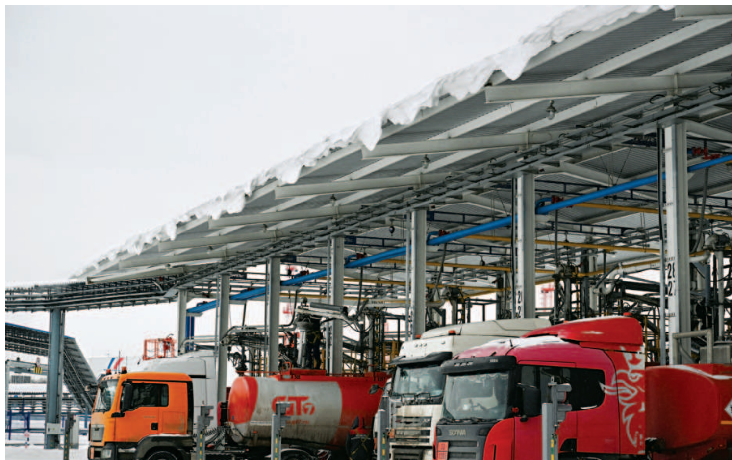
The photo taken on December 13 shows automated fuel loading systems at the grounds of a fuel tank farm of Russia's oil pipeline giant Transneft. Russia may produce between 515 and 538 million tonnes of oil next year, while exports will be broadly unchanged, at 250 million tonnes.
