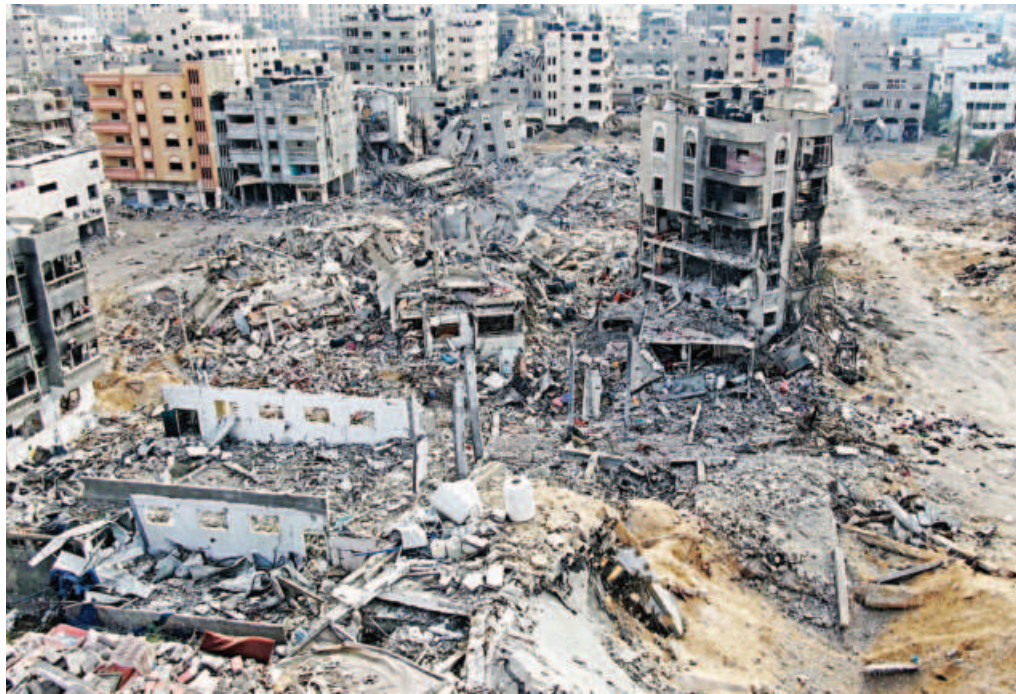
An aerial view shows destroyed buildings in Beit Lahia following Israeli bombardments in the northern Gaza Strip yesterday.
