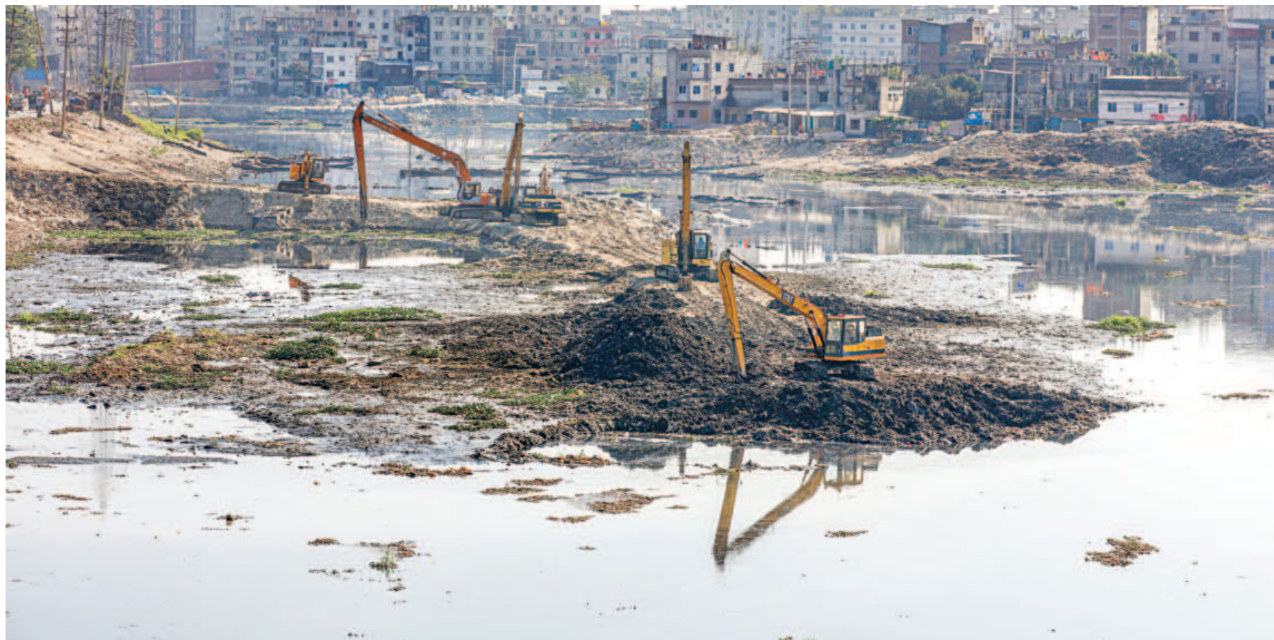
Dhaka South City Corporation is excavating this old channel of the Buriganga in the city's Kamrangirchar area to restore the river's navigability. It will later carry out some beautification work along the banks.
