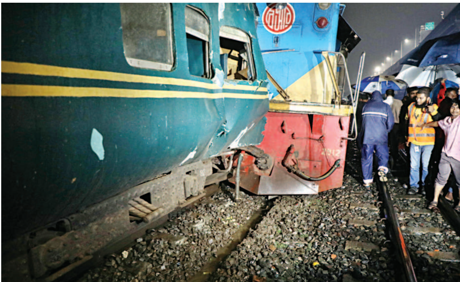
The locomotive and a carriage of Titas Commuter train derailed under the Dhaka Elevated Expressway near Tejgaon Railway Station yesterday evening after the train hit a crane being used in the construction of the expressway as the latter was crossing the rail track. The accident snapped rail communication between Dhaka and the rest of the country for five hours from 5:00pm.
