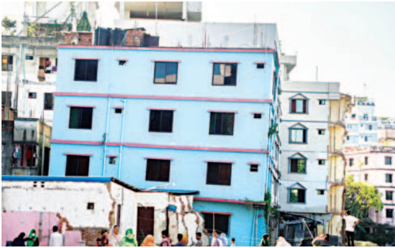
Residents of five buildings in Shahid Nagar of Chattogram city’s Bayazid area were evacuated after a building in the area tilted during re-excavation work of a nearby canal on November 25. PHOTO: RAJIB RAIHAN
