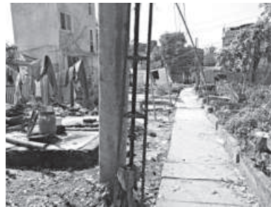
This walkway and structure were set up on a canal.
