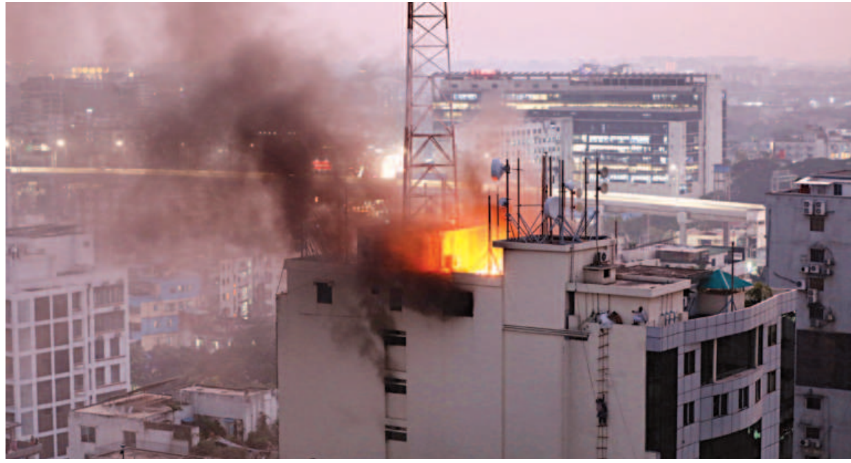
A fire broke out on the 12th floor of the 14-storey Khawaja Tower in Dhaka's Mohakhali area yesterday afternoon. Eleven units of the Fire Service and Civil Defence were working to douse the flame and rescue those trapped inside the building.
