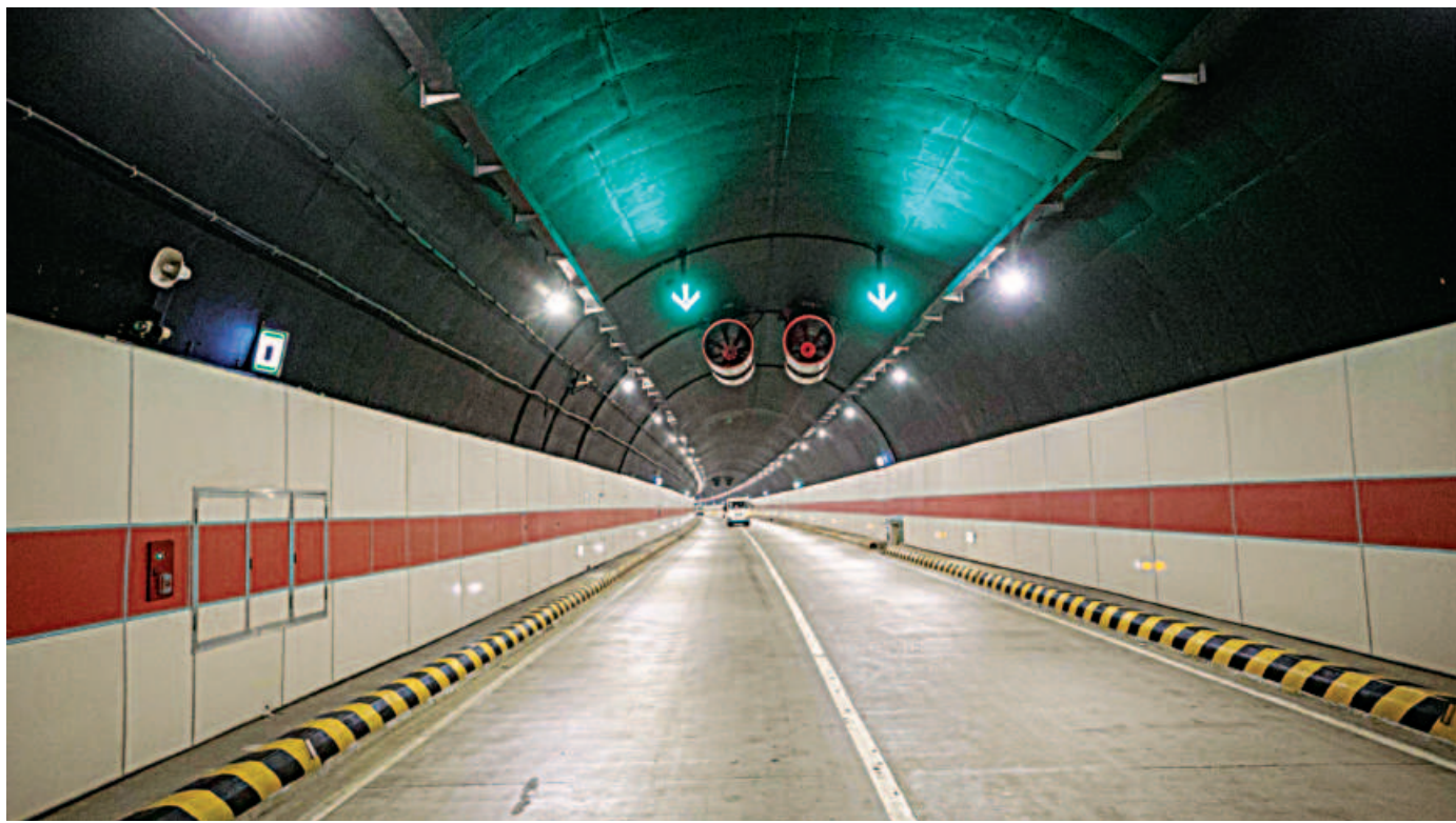
The Bangabandhu Sheikh Mujibur Rahman Tunnel under the Karnaphuli in Chattogram. Prime Minister Sheikh Hasina is to inaugurate the country's first tunnel tomorrow. The 3.31km tunnel will help improve road communication with Cox's Bazar and Bandarban.
