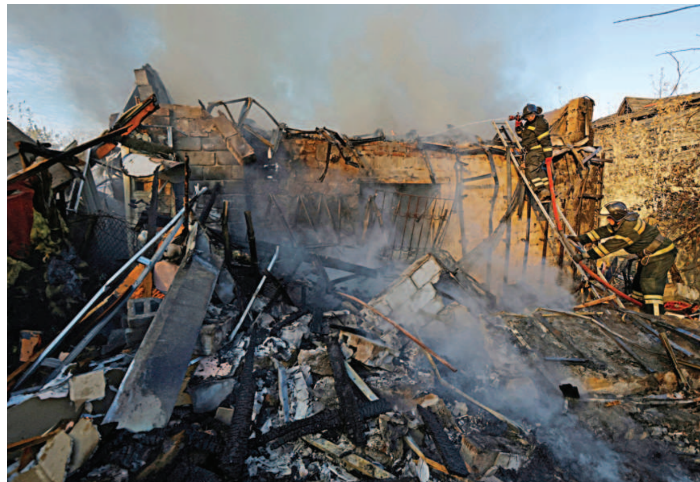
Firefighters work to put out fire at a house that was hit by shelling in the course of Russia-Ukraine conflict in Donetsk, Ukraine yesterday.
